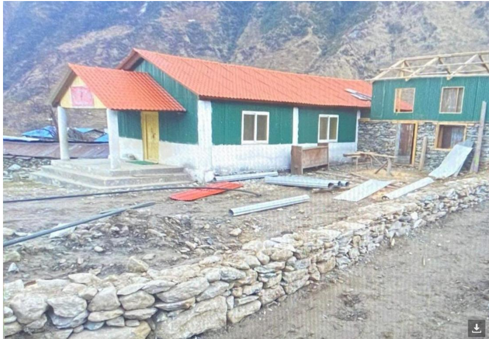
Lapdung Church Building (Nepal) with new addition under construction
